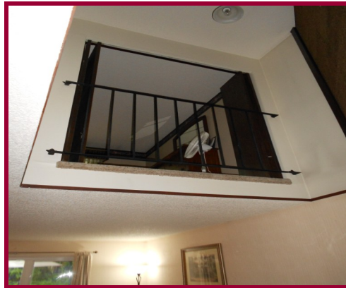
View From 1st Floor Entry
