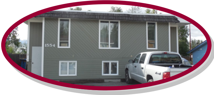
Front of Building
