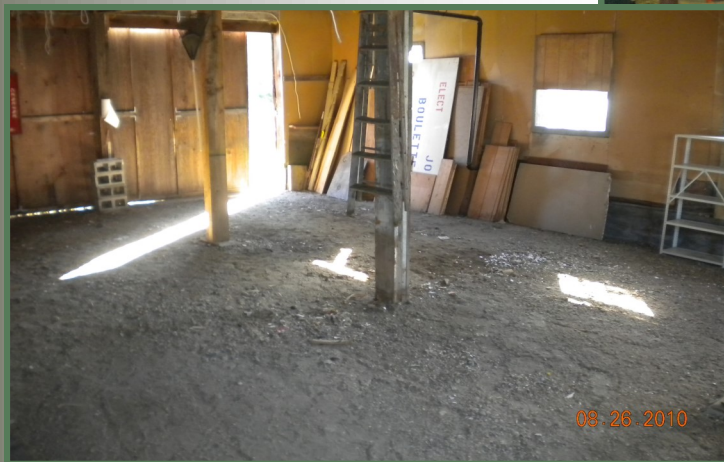
Unheated attached garage
